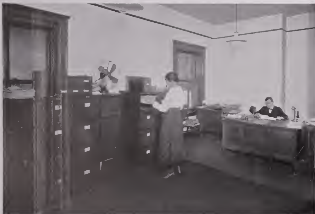
OFFICE OF TRAFFIC MANAGER First National Bank Building
